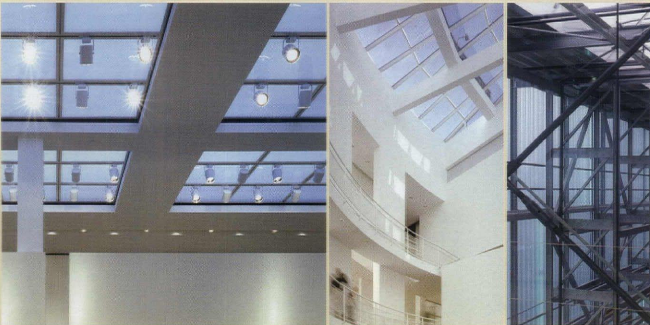
Daylighting is an integral component of many projects recently published by Architectural Lighting . Left to right: A laylight complements track lighting at the Racine Art Museum (September/October 2003). The High Museum's atrium skylight originally allowed too much sunlight into the galleries; window films and shades solved the problem (January/February 2004). An industrial U-glass provides daylight to the interior of Erco's warehouse and an interesting texture to the exterior (September/October 2003). Photographers, left to right: Chris Barrett/Hedrich Blessing; Jonathan Hillyer; Jörg Hempel Photodesign.
