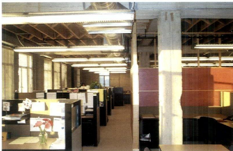
The American office in the new millennium: the drop ceiling is gone and the metal fixtures are exposed. For linear pendants, the trend is toward a more prominent downward component.
