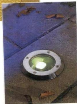
FIBER OPTICS ARE PROVIDING THE UPLIGHTS ON THIS BUILDING. WITH A TOTAL EQUIPMENT COST OF LESS THAN $400 PER FIXTURE, THIS JOB COMPARES FAVORABLY WITH CONVENTIONAL UPLIGHTS. PHOTOS COURTESY OF VISUAL LIGHTING TECHNOLOGIES.
