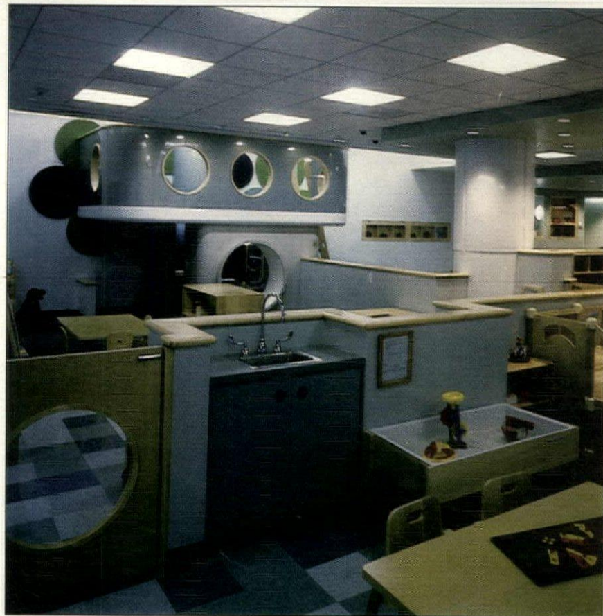
A MIX OF FLUORESCENT 2-FT X 2-FT. CEILING FIXTURES AND DIMMABLE RECESSED INCANDESCENT DOWNLIGHTS PROVIDE AMBIENT ILLUMINATION IN THE CENTER. THE DOWNLIGHTS MAY BE DIMMED DURING NAP-TIME QUIET ZONES AND THE FLUORESCENTS PROVIDE GLARE-FREE ILLUMINATION.
