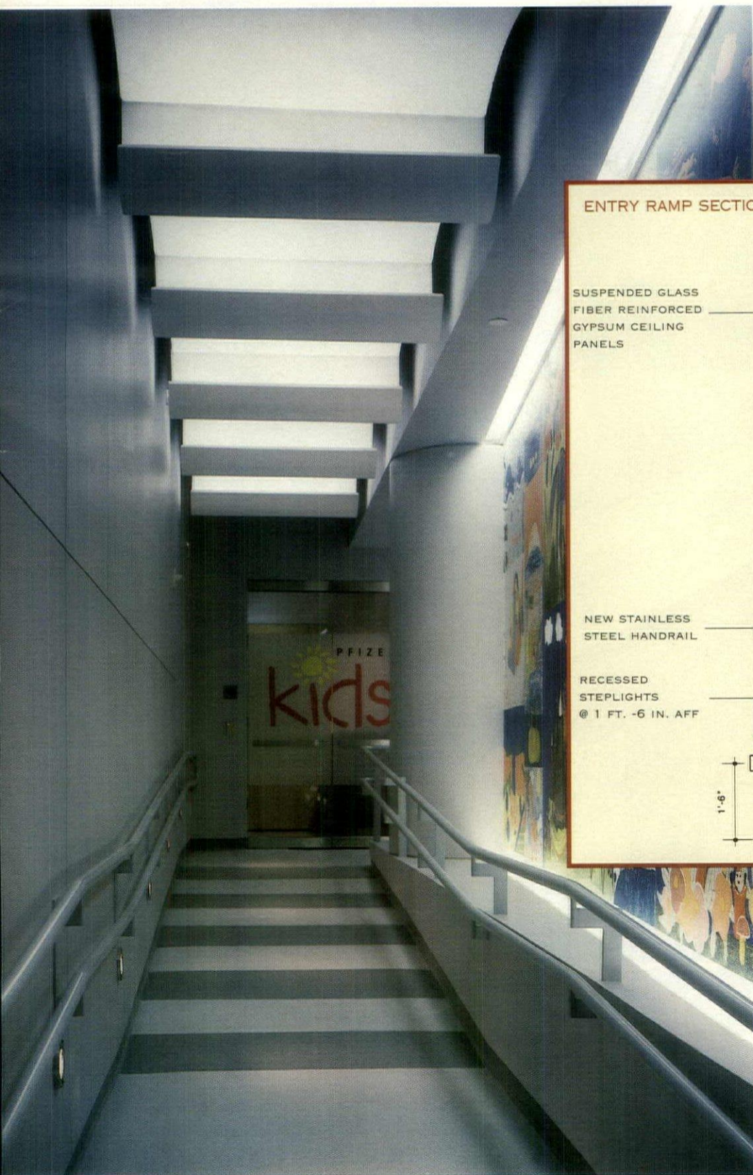
LEFT & OPPOSITE: IN THE 40-FT.-LONG CORRIDOR LEADING TO THE CHILDCARE CENTER, A SERIES OF UNDULATING CEILING PANELS MADE OF REINFORCED PLASTER ARE ILLUMINATED WITH INDIRECT FLUORESCENT LIGHT AND DRAW VISITORS TOWARD THE ENTRANCE. COVES FITTED WITH CONTINUOUS FLUORESCENT T8S ILLUMINATE A FLOOR-TO-CEILING MURAL OF CHILDREN'S ARTWORK FROM ABOVE AND BELOW.
