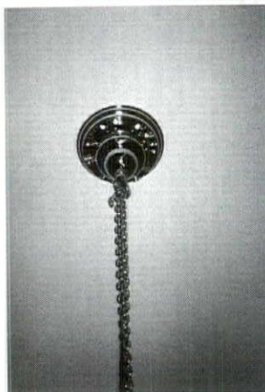
Conservation Lighting Tech.'s units hidden in stem base.
