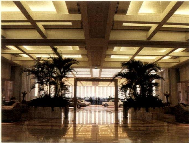
Main lobby ceiling shows the grid system of recessed fluorescent and incandescent lighting.
