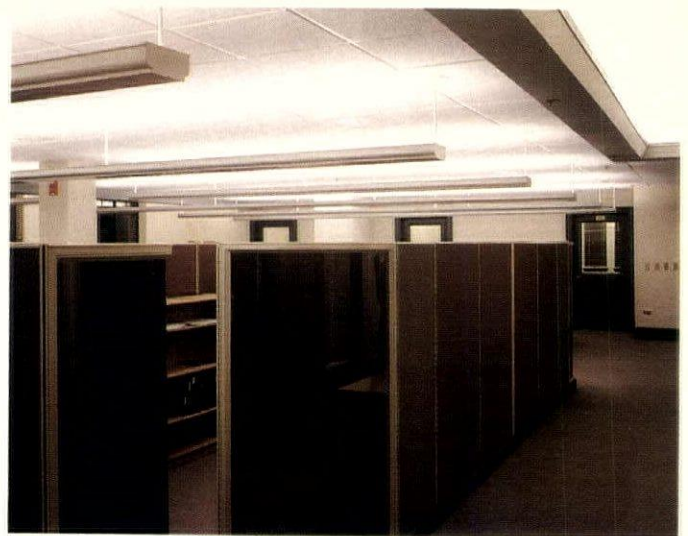
Interior of renovated office space showing custom indirect fluorescent luminaires and built-in light cove.
