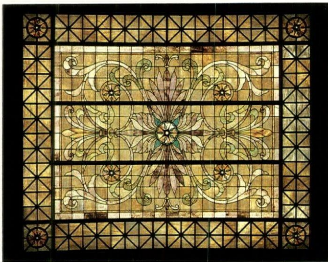
Restored skylight in center of lobby.
