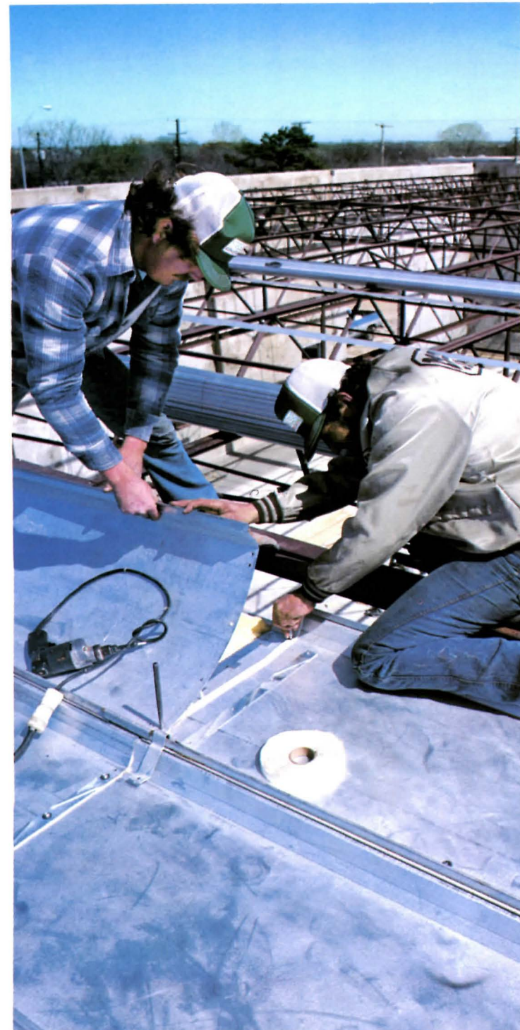
Vulcraft's unique pre-punched, pre-notched end lap assures proper installation and weathertightness.
