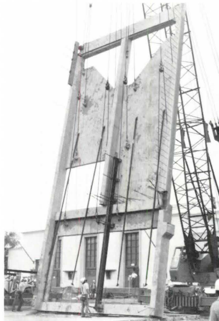
Top, entrance to the sports pavilion from the shorter right side of the plan above. Right, a crane tilts a wall panel into place. Across page, light and color enliven the interior, its windows creating the illusion of a floating roof.
