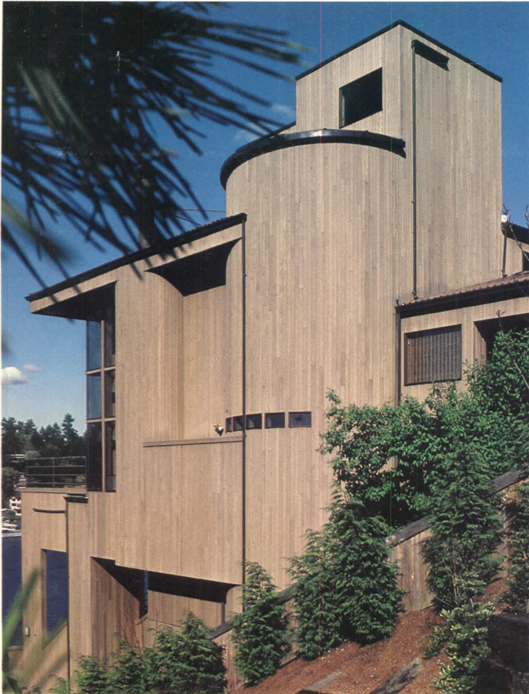
Architect: Paul Steven Myrwan, AIA, Seattle, Washington.
