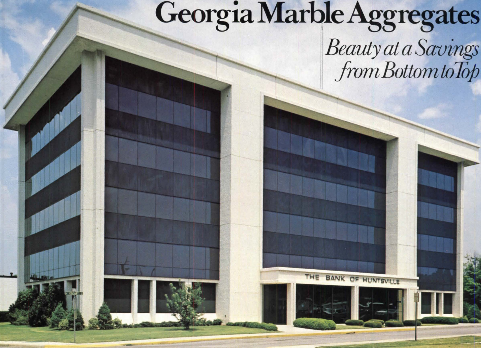
The Bank of Huntsville, Huntsville, AL./ Design & Construction: Bank Building Equipment Corp., St. Louis, MO. Specialty Contractor: Acousti Engineering of Alabama, Birmingham, Huntsville and Dothan, AL. Material: Georgia White.
