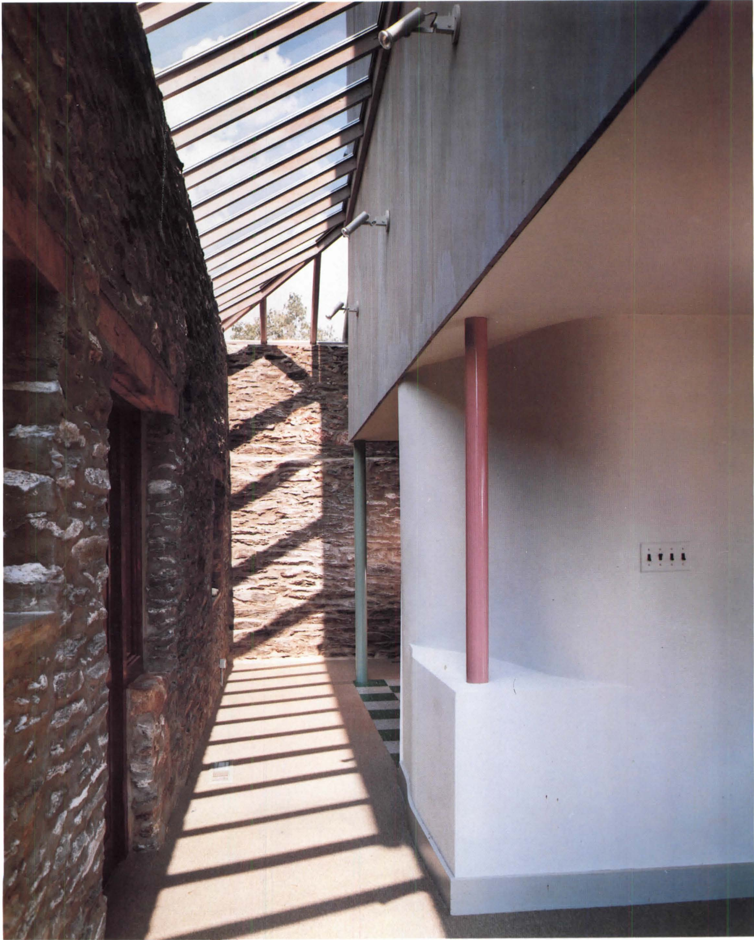
Linking the old foundation wall, with entrance, and the new house is a plexiglass-covered corridor; in the attic-study (across page), a stair with Corbusian rail rises through an angled slot. The room is multi-colored but muted and proportions are in miniature.
