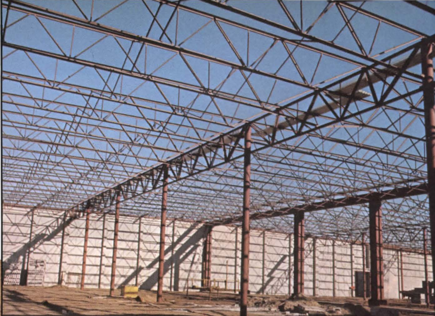
Economy results from high strength to weight of steel joists and joist girders. More efficient design and erection of primary structure is possible because fewer columns and beams are needed.
