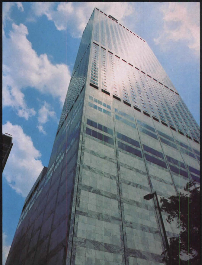
Water Tower Place, Chicago, Ill. | Arch: Loeb, Schlossman & Hackl
