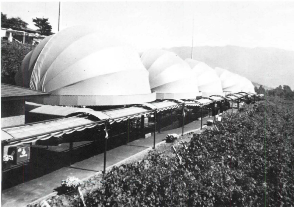
Fabric Roofing: The 1979 international achievement award for "new and unusual designs and applications for industrial fabric" was awarded by the Industrial Fabrics Institute to Taiyo Co. Ltd. of Tokyo for a roof over an open air restaurant at the Suntory Yamanashi winery in Japan. A series of polyester fabric domes form the restaurant's only roof. Motorized, they open down the center, allowing diners to view blue sky or starlight. Entries were judged on concept, design and manufacture.
