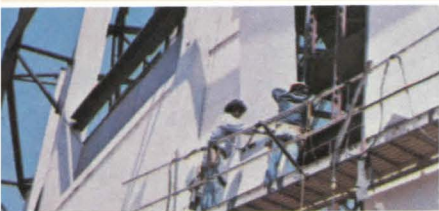
J-M panels were face mounted to steel studding, requiring about 25 per cent less installation time than conventional masonry techniques.
