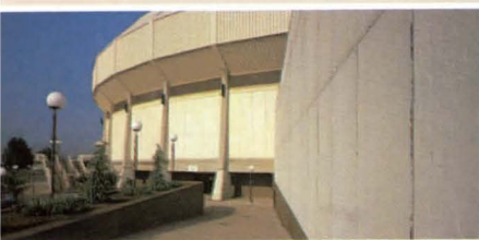
Stonehenge architectural panels cover 95 percent of the exterior of the Center, providing an attractive, stonelike appearance that will not change due to climate conditions.
