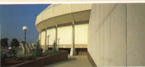
J-M Stonehenge architectural panels cover 70 per cent of the exterior of the Center, providing an attractive, stonelike appearance that will not change due to climate conditions.
