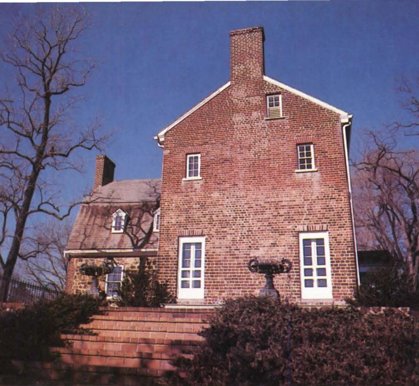
Belvoir in profile, with the original cottage structure at left.
