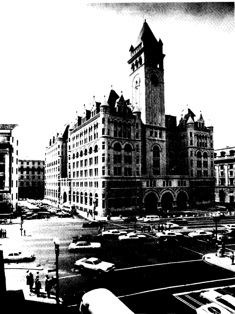
Above, the old post office meets the unfinished Internal Revenue building. At left, a fountain on the edge of the so-called great plaza gives a clue to unfulfilled landscaping plans. The paved area has been crowded with cars since the 1930s.
