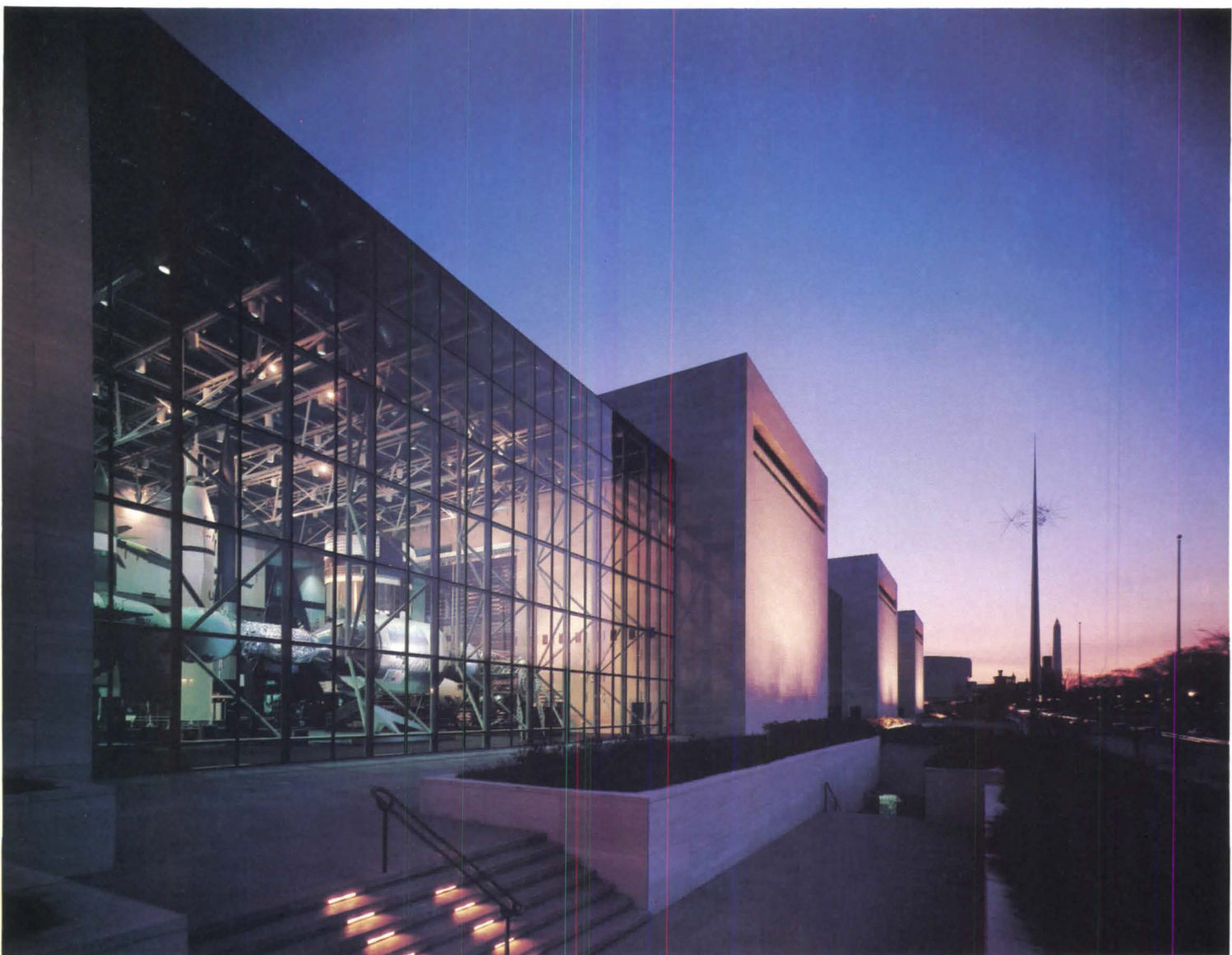
Full-height glazed panels expose the flying machines of the 1976 Air and Space Museum, by Hellmuth, Obata & Kassabum, to the Mall.
