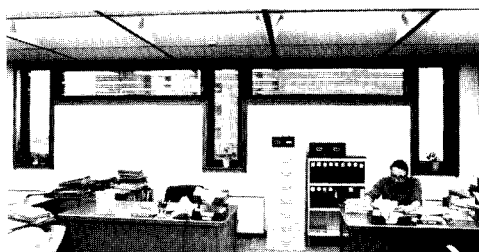
Blinds are encased between two panels of glass and thus inaccessible in case of malfunction. Below, the second floor with its additional horizontal windows.
