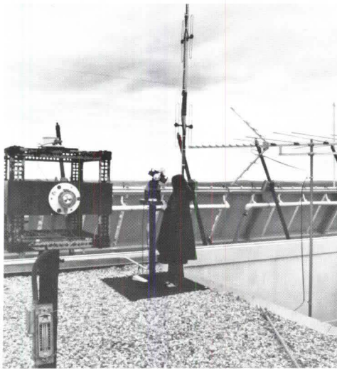
Rooftop appurtenances: solar collectors and a weather-monitoring 'sentinel.'
