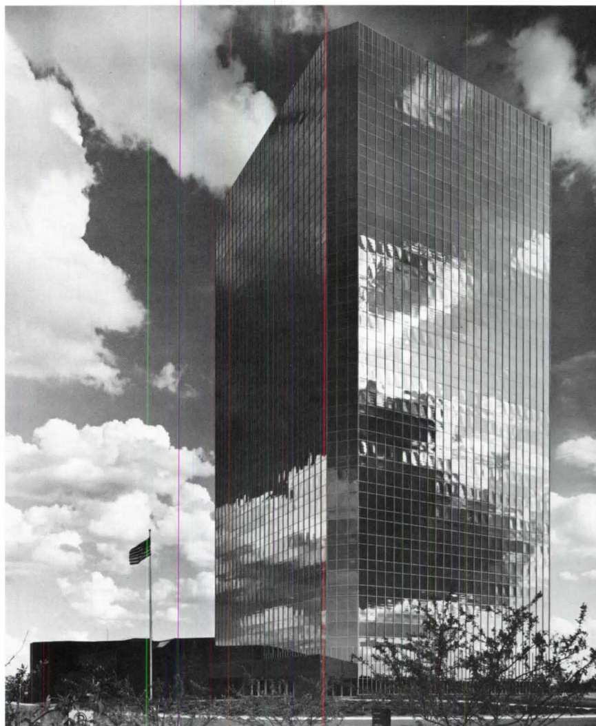
Truncated corners of tower add interest to square format chosen to conserve energy.
