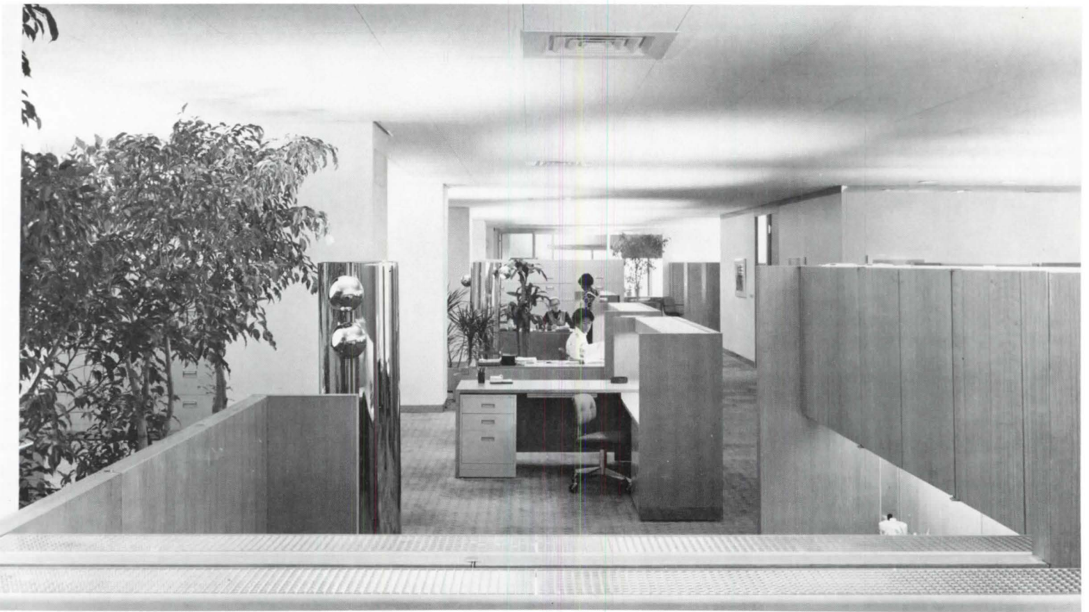
Atlantic Richfield's Philadelphia headquarters office lighting system has served as prototype for T/A illumination. Developed by Sylvan Shemitz, it reportedly delivers 2.56 watts per square foot.
