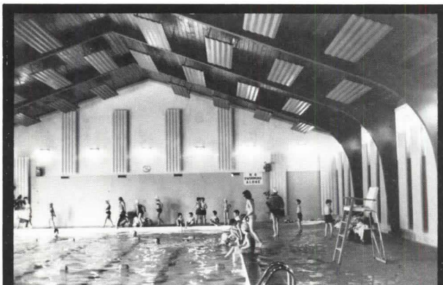
EFPs used for acoustic treatment at YMCA Pool, Danvers, Mass.
