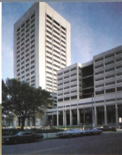
Cuyahoga County Justice Center. Cleveland, Ohio. Exterior: ASG Bronze. Interior: ASG Penal-Gard and Bullet Resisting glass.
