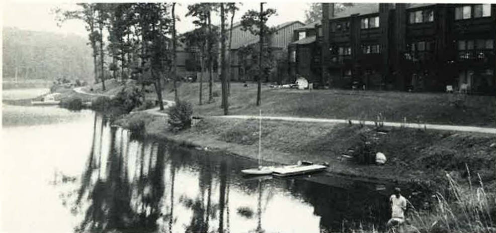
Industry along I-270 and a Germantown residential development.
