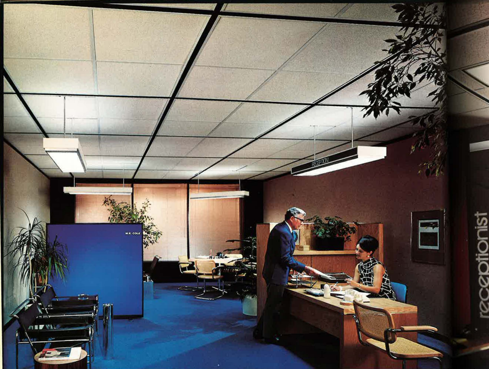
This pendant fixture, movable to many points in the room, provides both quality task lighting and substantial energy savings.
