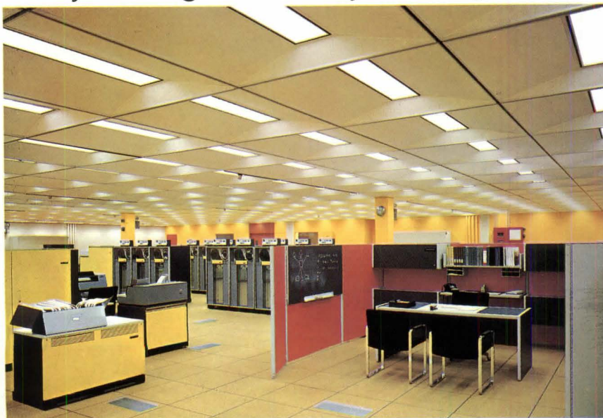
Datacenter/The Equitable Life Assurance Society of the United States, Easton, Pennsylvania, Architects: Kahn and Jacobs, New York City, Ceiling System: Armstrong C-60/60 Luminaire
