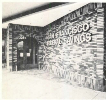
San Francisco Federal Savings; Valley Fair Shopping Center, San Jose, California. Hawley and Peterson, Architects.
