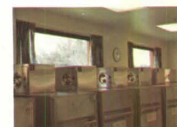
Big Carda Teak windows in a hospital kitchen
