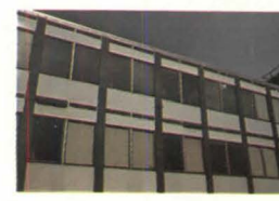
Teak windows in metal wall. Installed in 1961
