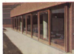
Massive Teak sliding doors
