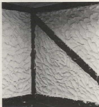
Highly textured finish coat achieved with sponge.
