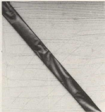
Scratch coat of white Thoroseal Plaster Mix over brown coat.
