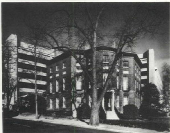
A blend of old and new. A graceful expanse of reinforced concrete harmonizes with the 18th century Octagon House.
