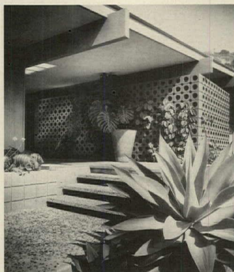
Small private exterior areas are important yet inexpensive (top left); special cast concrete block adds privacy and interest to the entrance (bottom left); simple plastic bubbles are a source of interior light (above).
