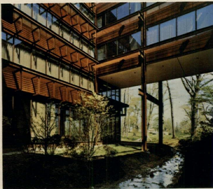
Weathering Steel grating at each floor level, between the exterior walls and the sun screen, facilitate washing the bronze-tinted insulating glass.
