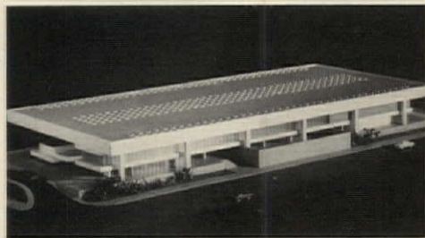
A model of an office for a textile association is the 1969 design of Vilanova Artigas.
