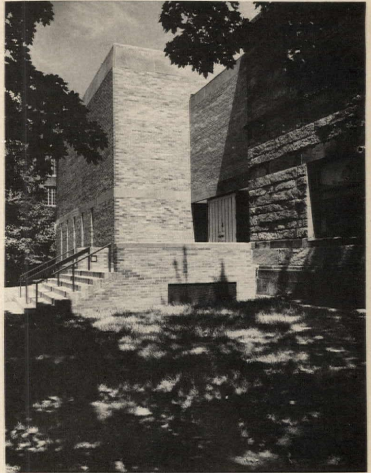
Huygens & Tappé Inc.: Concert Hall and Library, Longy School of Music, finished in 1970 in Cambridge, Massachusetts.
