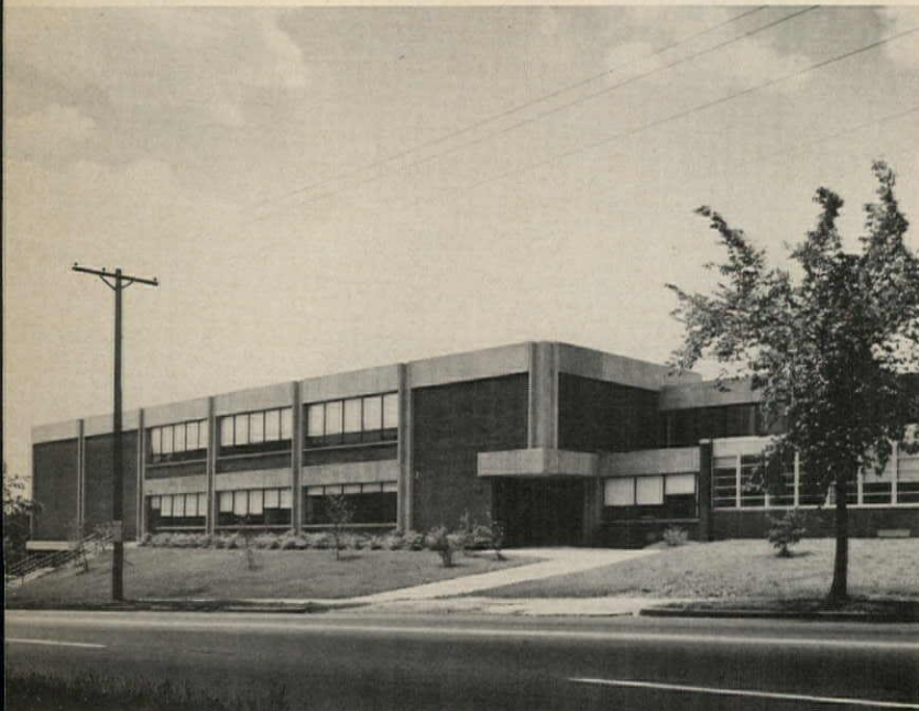
Webb Elementary School Addition (above), which has a stilted second floor to conserve scarce play place, is one of the District's first public schools with open planning. Nalle Elementary School Addition (below) is planned to integrate with the original school both functionally and in appearance. The Georgetown Day School (across page) is a private school whose playtower, also designed by the Bryant & Bryant firm, is of differing levels and shapes of openings leading to balconies. The upper level can only be reached by a rope. Kids love it.
