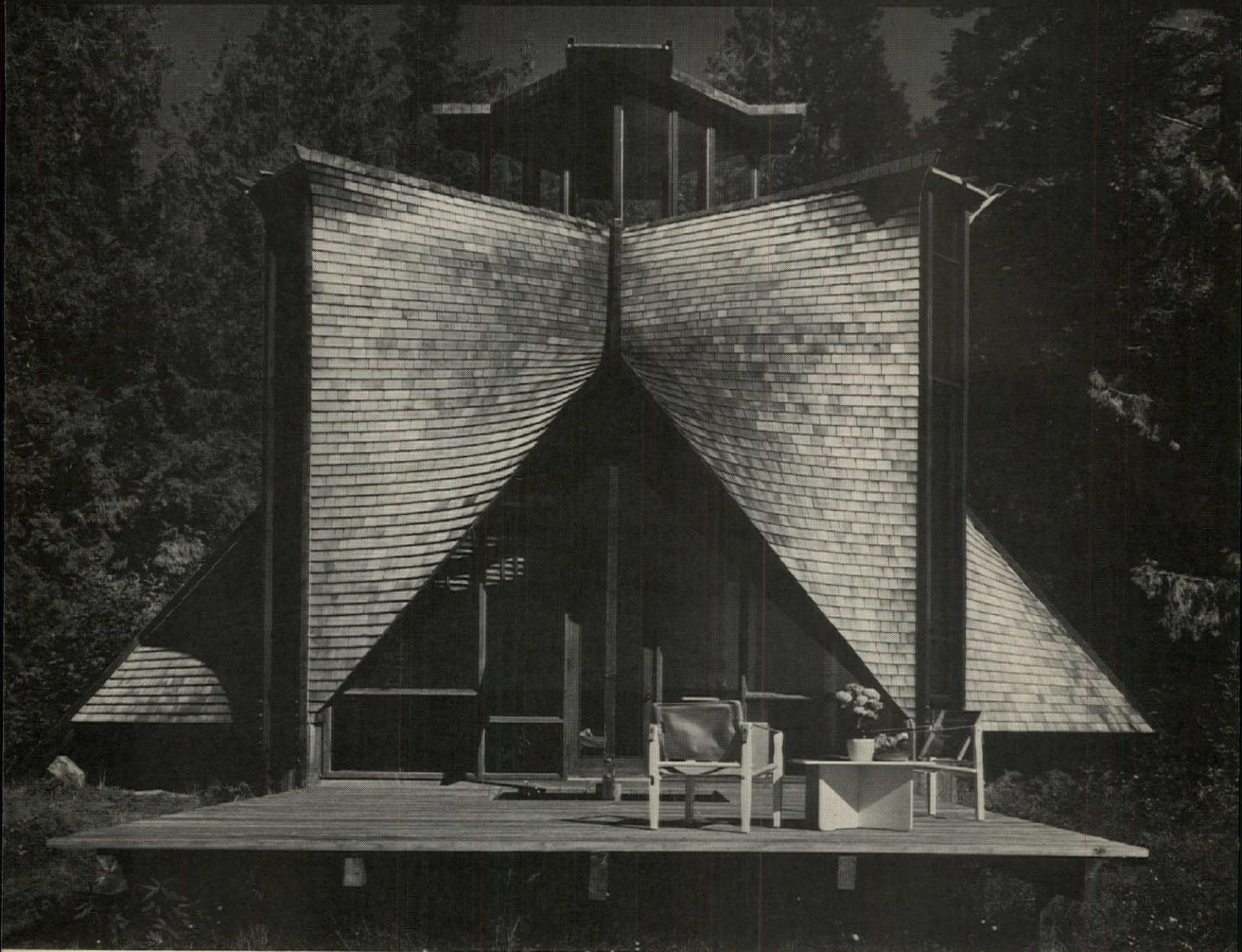
Vacation home, Hood Canal, Washington. Certigrade shingles No. 1 Grade, 16" Fivex. Owner/Architect: Robert E. Cooper.
