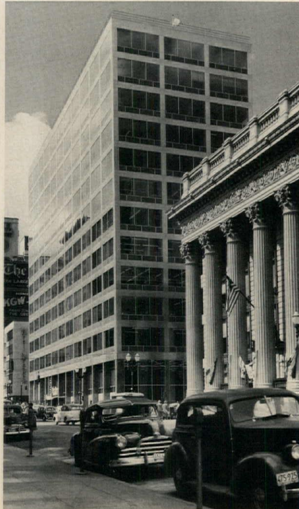
The first wing of the Portland Art Museum, opened in 1932, gave national recognition to Belluschi (left). The block was recently completed by him in collaboration with Wolff, Zimmer, Gunsul & Frasca. The Equitable Building in Portland (right) is a tower of green glass and aluminum. It was the first of its kind built in the US.
