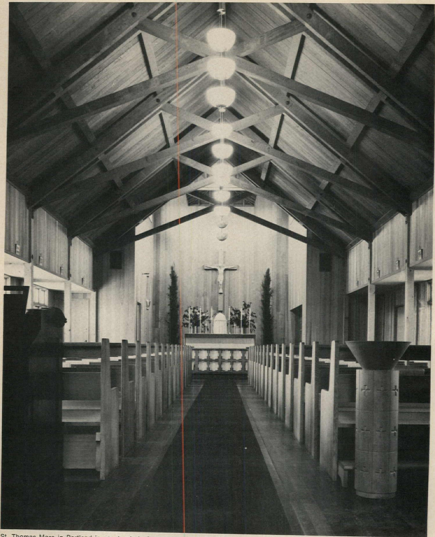
St. Thomas More in Portland is constructed of wood both within and without. Its scissors trusses open inside. Designed in 1939, this church was the first to come from Belluschi's office, starting a worthy tradition.
