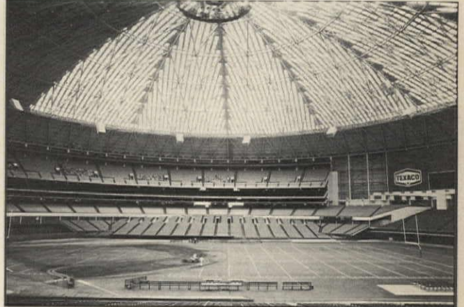
The Astrodome, 1965. Architects: Wilson, Morris, Crain & Anderson; associate architects: Lloyd & Morgan
