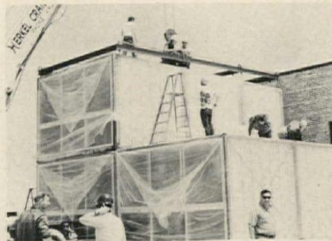
Stacking space modules for a five-story motel.
