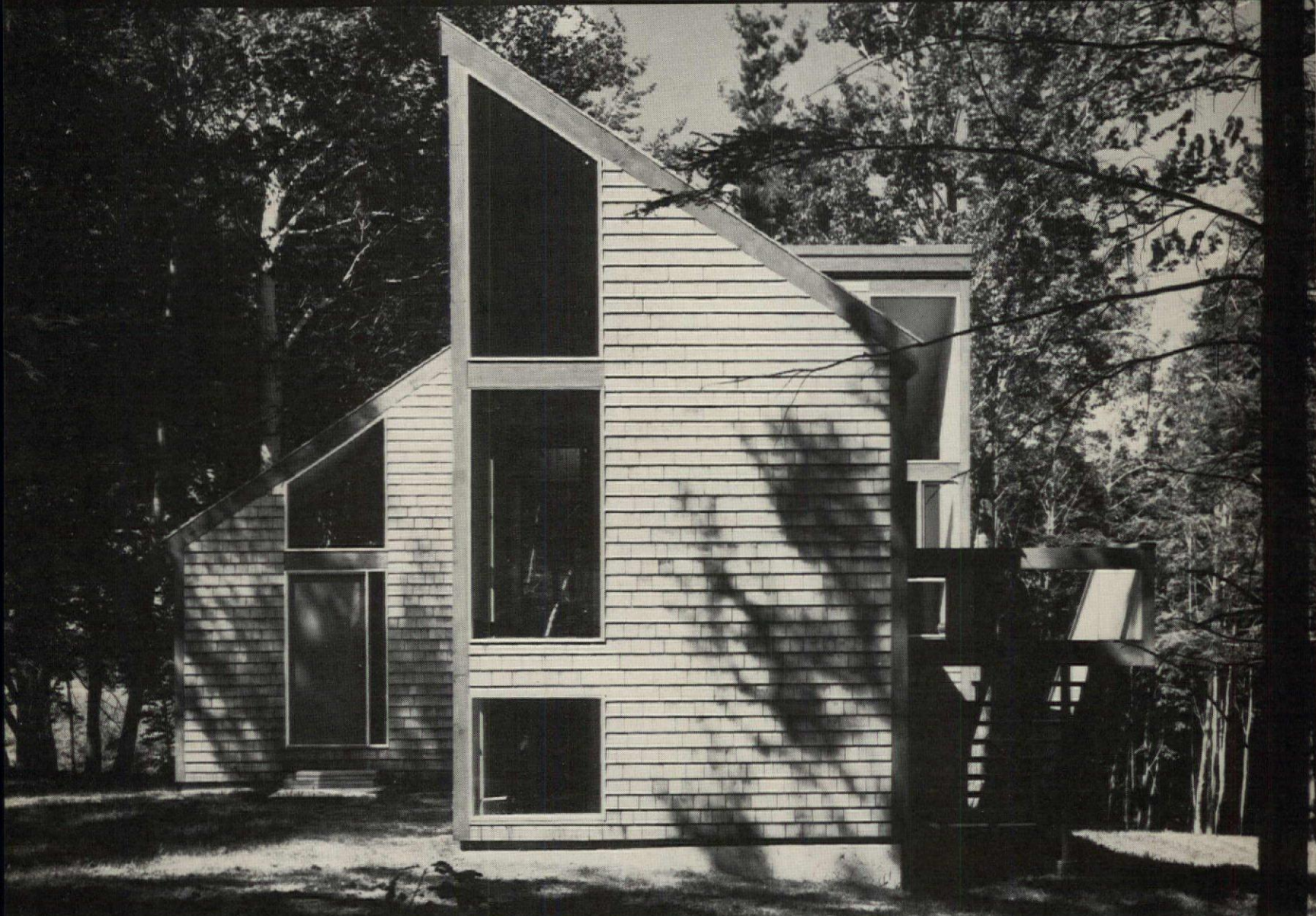
Vacation home at Franconstown, New Hampshire. Certigrade Shingles No. 1 Grade 16" Fivex. Architect: Brett Donham.
