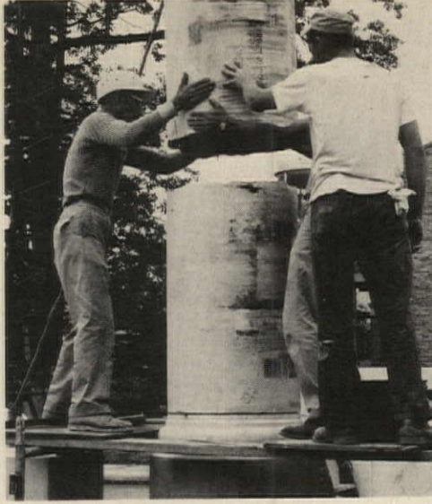
Stonemason sets first stone in April 1965, supervises placement of a section of a column and smooths one of the more than 7,000 numbered stones.
