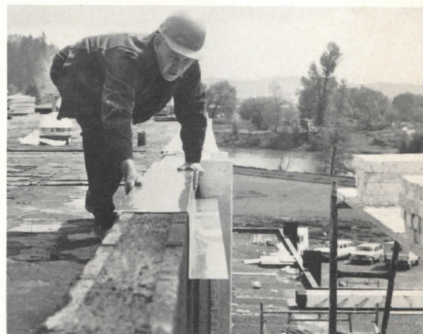
Pre-formed flashings were easily positioned prior to joining.
