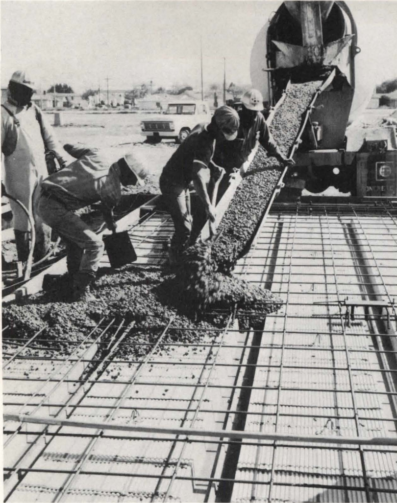
Brickplate face down in forms with mastic sealing back of joints, steel reinforcing in place and concrete being poured; panels being erected and secured in place. Tanforan Shopping Center, San Bruno, California.
