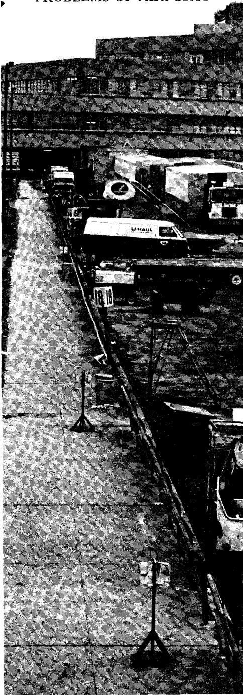
Nineteen mobile classroom units put together end to end keep passengers from three airlines out of the weather at Greater Philadelphia Airport during construction of new terminal. Robert M. Ovelman, director-facilities of Allegheny Airlines, designed the instant terminal over a 600-foot walk. With wheels off units, dividing walls removed and carpet installed, presto: business as usual. Total cost was $300,000, work took less than one week, units can be used again.
