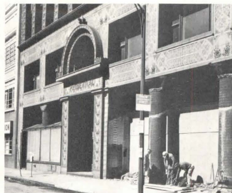
Modernization continues at Prudential, but Sullivan's ornamentation is preserved.
