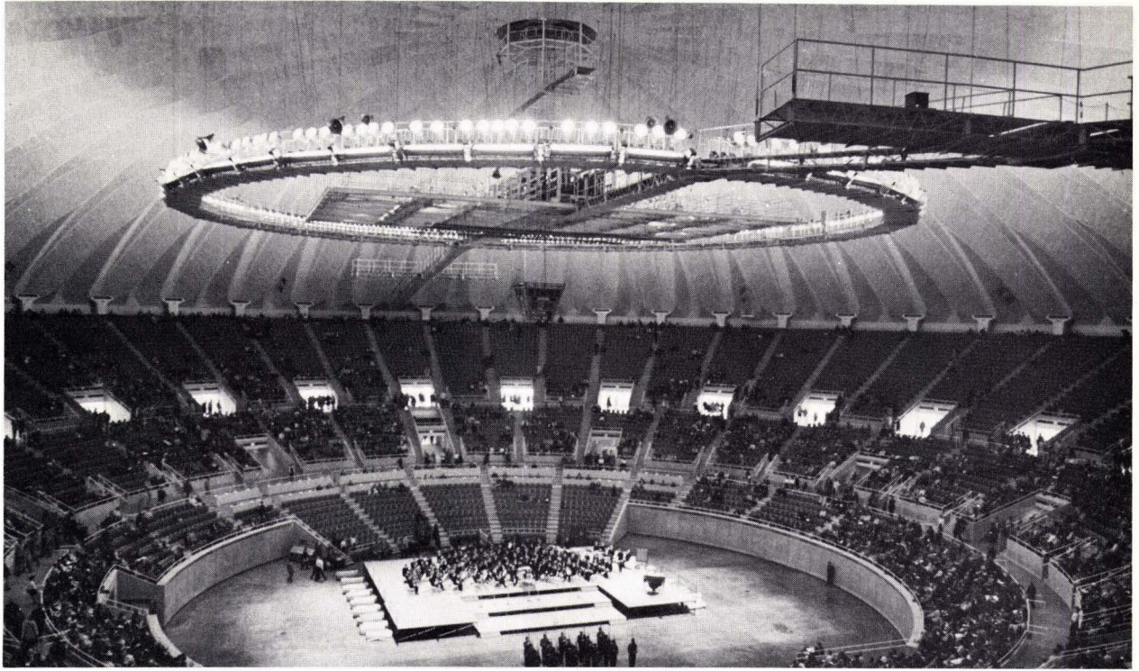
Assembly Hall, University of Illinois, Urbana. Architects: Harrison & Abramovitz.
