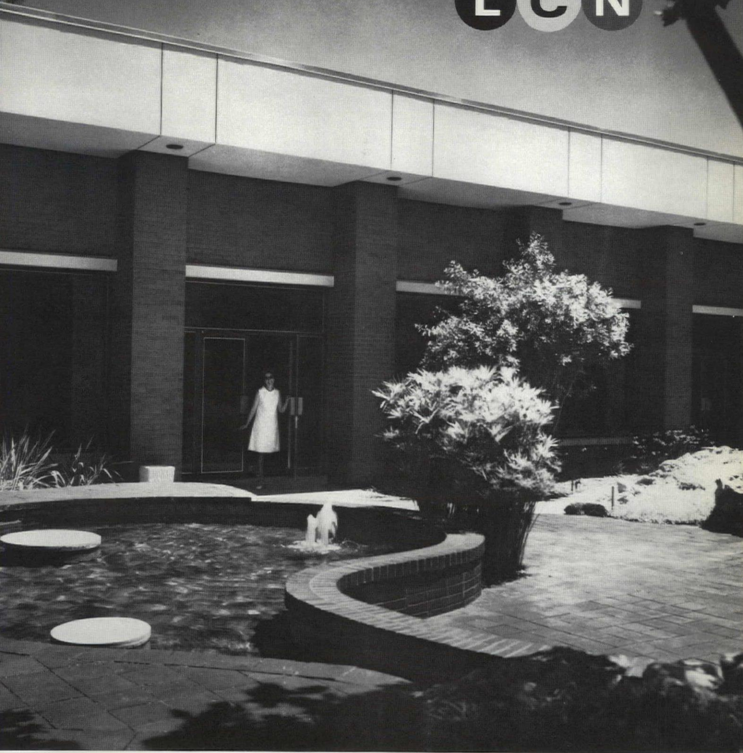
Overseas Operating Center, American Telephone and Telegraph Company—Long Lines Department, Jacksonville, Florida. Reynolds, Smith and Hills, Architects—Engineers—Planners; Jacksonville.
