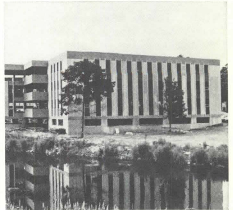
Over-all view of structure reveals pleasing contrast between Ace Corspan panels and Ace Colorlith ® window spandrels.
