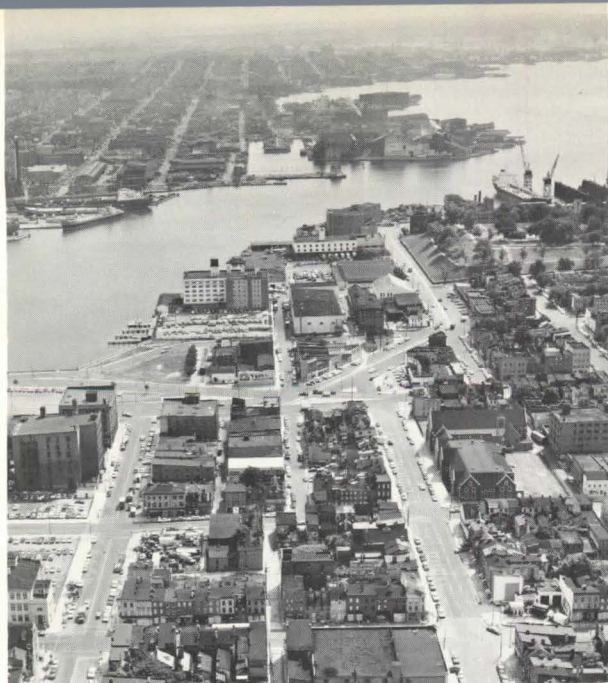
Baltimore's Inner Harbor as it looks today, a residential/business district including Federal Hill, right. Models, by Skidmore, Owings & Merrill, show original plan for
