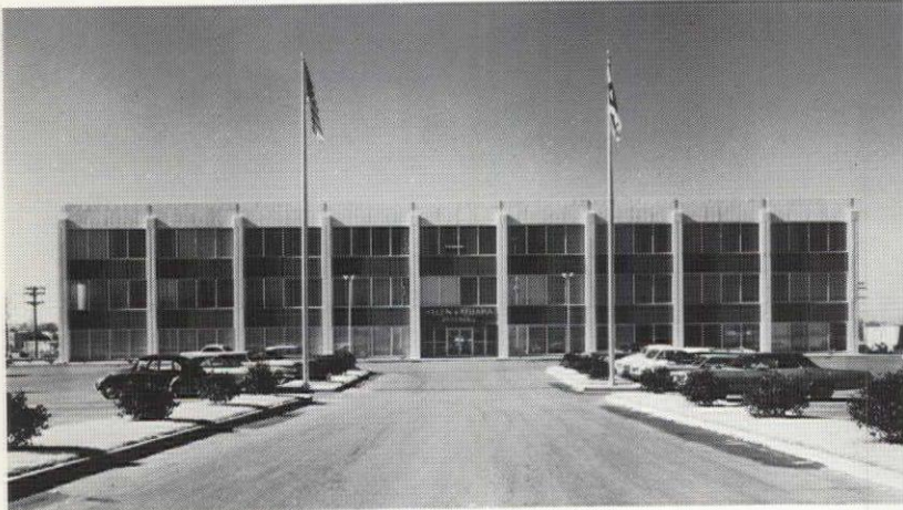
ALLEN & O'HARA BUILDING, Memphis, Tennessee. Architects: Robert Lee Hall Associates, Inc. General Contractor: Allen & O'Hara, Inc. Three Dover Oildraulic Elevators installed by Dover Elevator Co.
