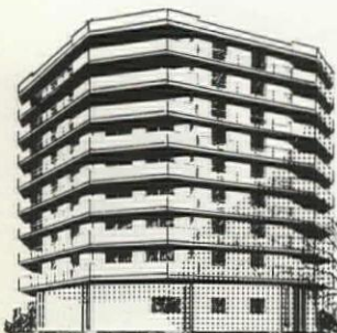
$5,525 saved in annual heating costs by Salem Towers Apartments in Malden, Massachusetts, with Temco Pre-Vent thru-the-wall Gas Furnaces in 80 apartments. Estimates for heating them electrically were $11,125 . . . compared with just $5,600 a year for the Pre-Vents.
