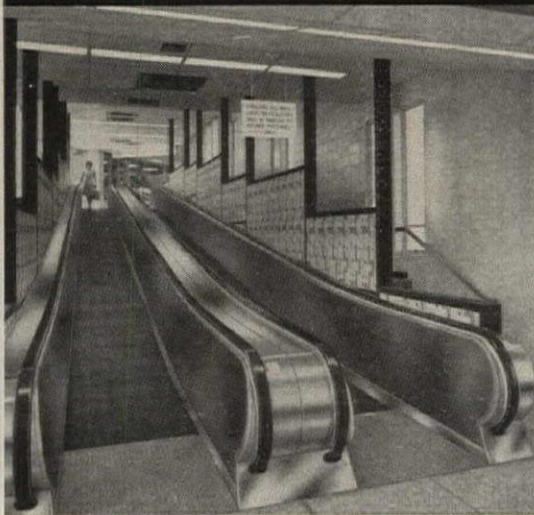
FOUR Montgomery POWER RAMPS at Stapleton have 40" tread width. Two Power Ramps have HORIZONTAL TRANSITION (horizontal entry — incline travel — horizontal exit.)
