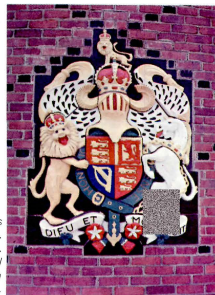
Old World Pavilion Group, Glass House Point, Jamestown, Va. Ballou and Justice, architects. Bas-relief cartouche and panel were custom-made in polychrome Terra Cotta.
