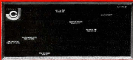
Alarm and Status Annunciator Panel
