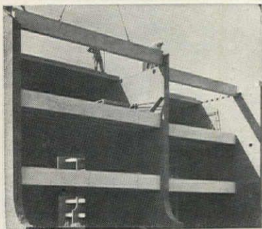
Floor system of precast concrete planks bears 4 inches on the masonry walls at Pennley Park. Precast concrete spandrel beams frame into the bearing walls to carry corridor and exterior panel walls. While floors are laid in one area, bricklayers erect walls in another. Utilities run through the corridors of the apartment project, whose bearing walls express the structural concept clearly.
