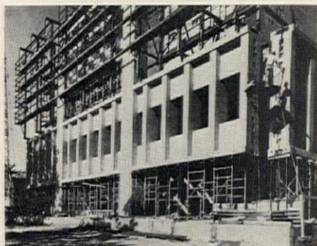
Precast Unprecedented: Sections of precast concrete are assembled on steel tendons by means of self-supporting monorail system and post-tensioned to form Vierendeel trusses. Design alternates truss and nontruss floors (right).
