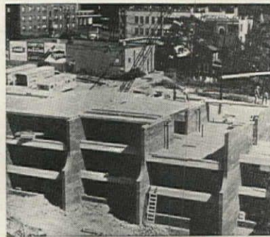
Floor system of precast concrete planks bears 4 inches on the masonry walls at Pennley Park. Precast concrete spandrel beams frame into the bearing walls to carry corridor and exterior panel walls. While floors are laid in one area, bricklayers erect walls in another. Utilities run through the corridors of the apartment project, whose bearing walls express the structural concept clearly.
