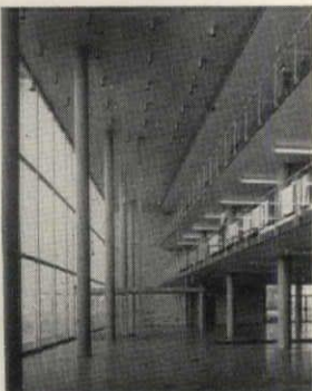
Dependable SONOTUBE Fibre Forms require minimum bracing and permit continuous pours as high as 40 feet.
