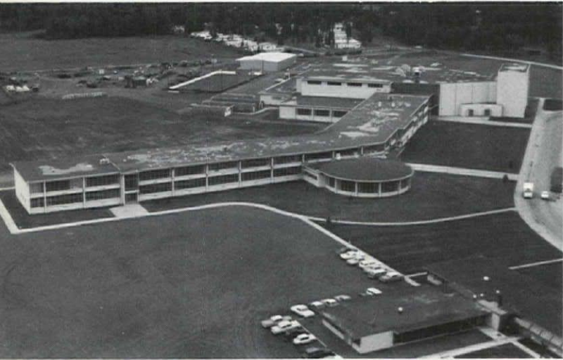
1 West Anchorage High School: relatively minor damage of circular library as compared to the adjoining classroom wing. 2 The city of Anchorage in the L-Street slide area: pile of rubble at left center contains the Four Seasons Apartments. Knik Arms Apartments is at top center. 3 West Anchorage High School: damage at the intersection of classroom wings and the corner of the gymnasium. 4 Cordova Building: damage to the lower part of the stair tower.
