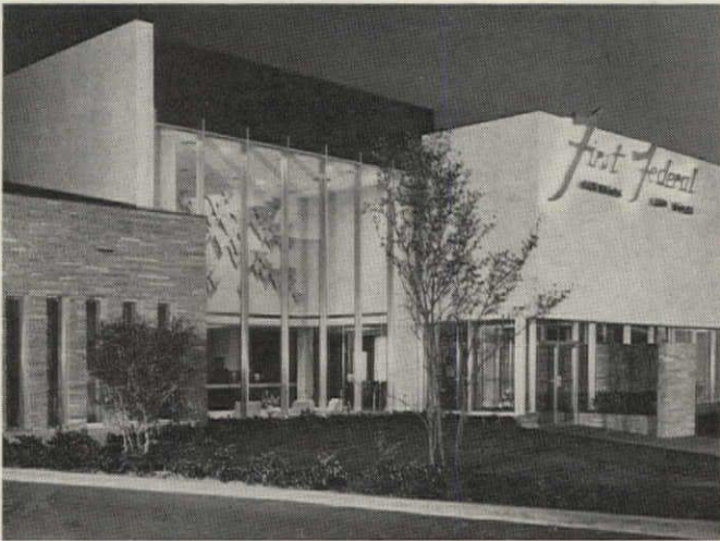
First Federal Savings & Loan — Wichita Falls, Texas / Architect: Bank Building & Equipment Corporation / Dealer: Southwestern Glass & Paint Company, Inc. / General Contractor: Bank Building & Equipment Corporation
