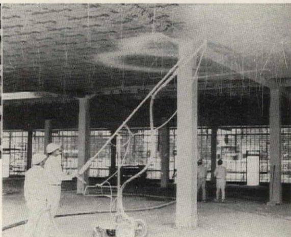
Fast machine plastering on K-LATH's GUN LATH.
