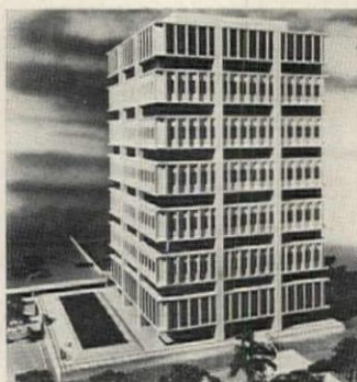
Precast Unprecedented: Sections of precast concrete are assembled on steel tendons by means of self-supporting monorail system and post-tensioned to form Vierendeel trusses. Design alternates truss and nontruss floors (right).
