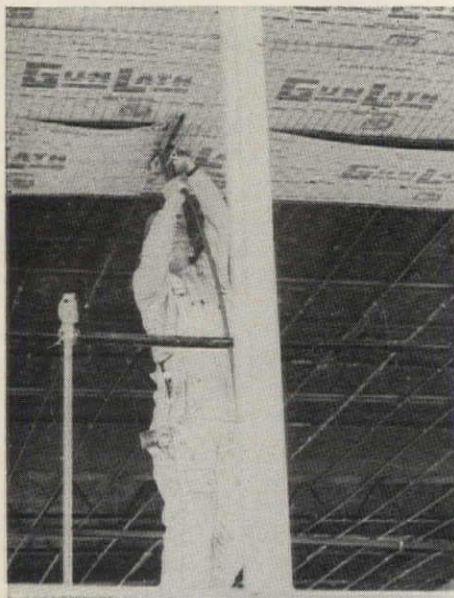
Mechanized lathing with K-LATH's GUN LATH.
