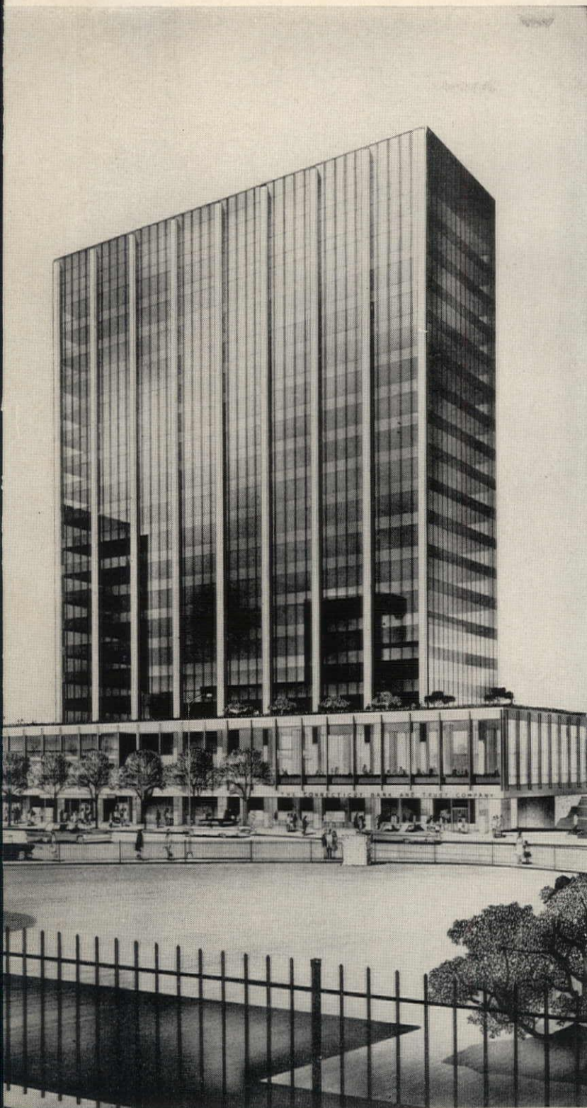
The Connecticut Bank & Trust Company, Hartford, Conn. Architects: Robert Allan Jacobs-Carson, Lundin & Shaw General Contractor: F. H. McGraw & Company
