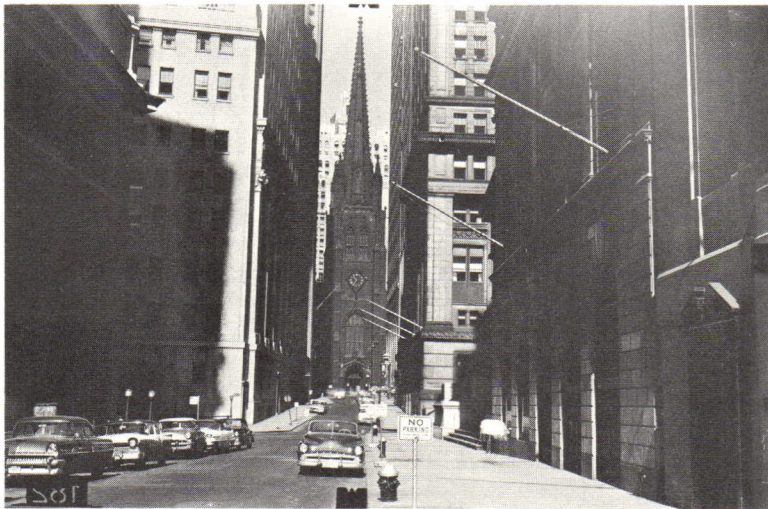
Stereopair of east façade of Trinity Church down length of Wall Street, New York City, September 1959. Wild T 30 Phototheodolite—inclination upwards 10.4g—base 22.68'—distance approximately 660'
