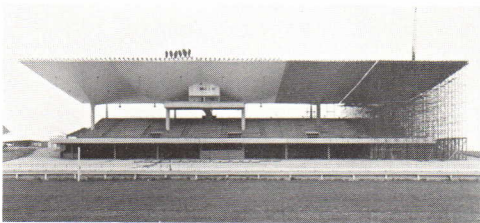
Scioto Downs, 6 May 1961. Second photo of a series recording settlement of hyperbolic paraboloid from which formwork is released
