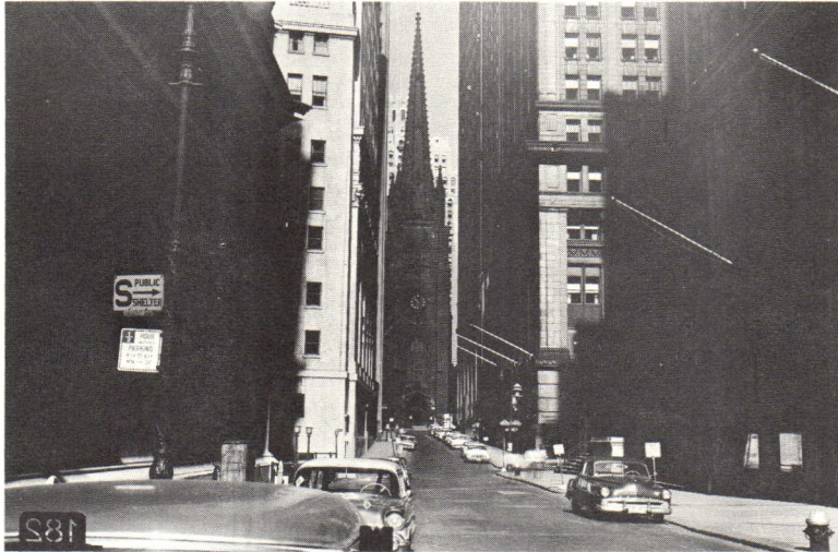
Stereopair of east façade of Trinity Church down length of Wall Street, New York City, September 1959. Wild T 30 Phototheodolite—inclination upwards 10.4g—base 22.68'—distance approximately 660'
