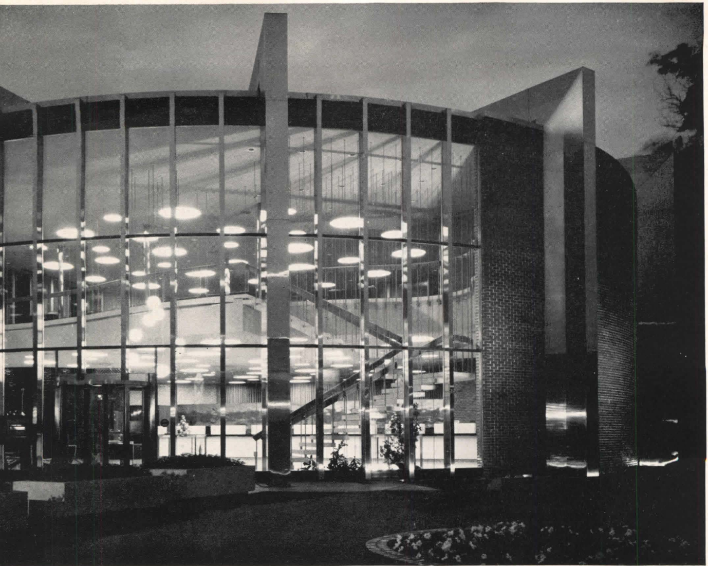
Stainless steel covered bents of this dramatic circular building serve as both structural and design elements. In secondary photo below, stainless steel rods from floor and ceiling hold treads of this distinctive floating stair in place.
