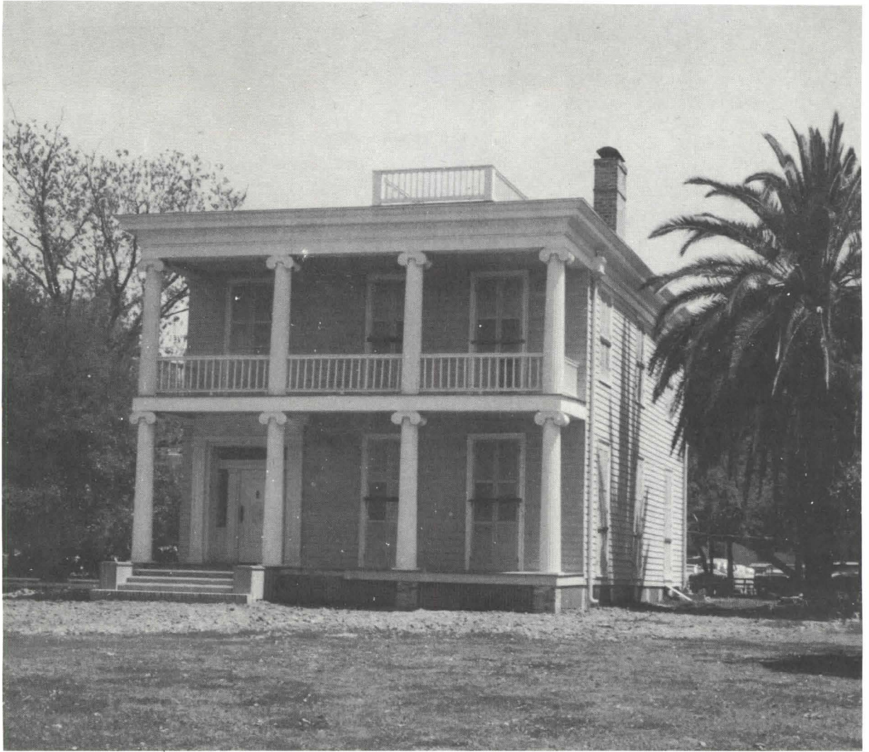
Nichols-Rice House after moving and restoration
