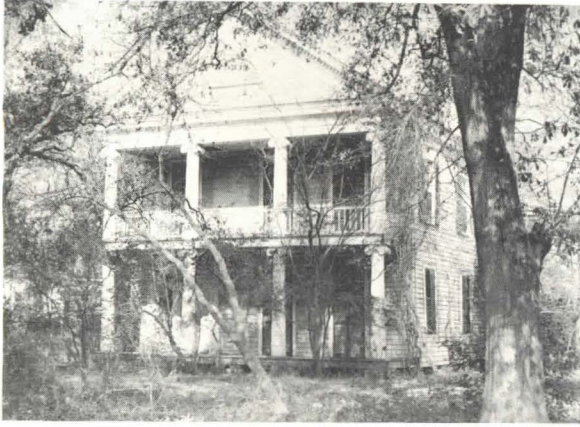
Above, before dismantling and moving. Note heavy later gable. At right, Greek Revival entrance doorway
