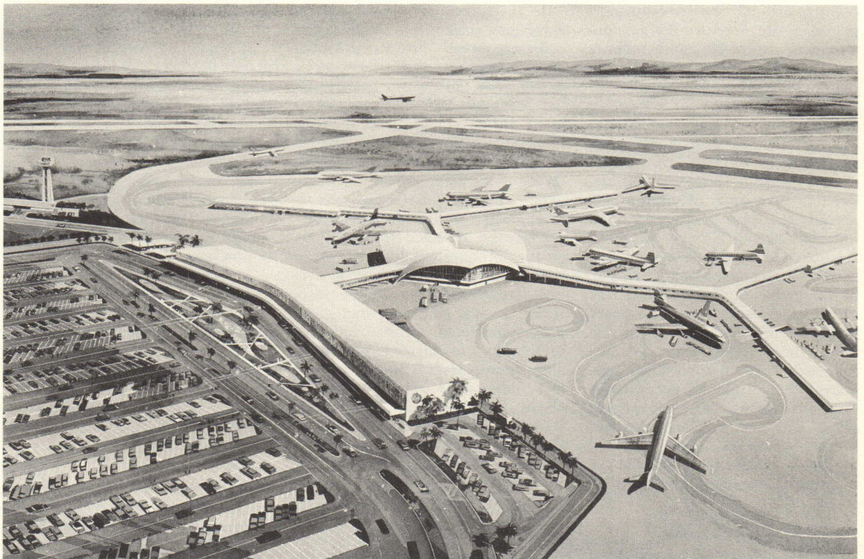
Las Vegas Airport, McCarran Field, Clark County, Nevada. Welton Becket and Associates, Architects and Engineers. Facilities for the $4,500,000 project will include: two primary two-story buildings (one for ticketing, baggage and airline offices; and the other passenger waiting terminal and restaurant: hexagonal, thin-shell ribbed concrete vault roof), passenger loading fingers (sixteen gate positions to accommodate largest jet airliners), control tower, fire station, and parking for 1400 cars. Complete passenger complex encloses 159,150 sf. Provisions for expansion to 24 jet positions by extension of fingers
