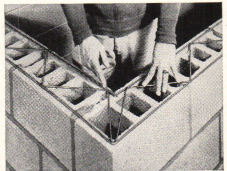
Two engineered products that meet a need. Dur-o-wal reinforcement, shown above, and Rapid Control Joints, below. Weatherproof neoprene flanges on the latter flex with the joint, simplify the caulking problem.
