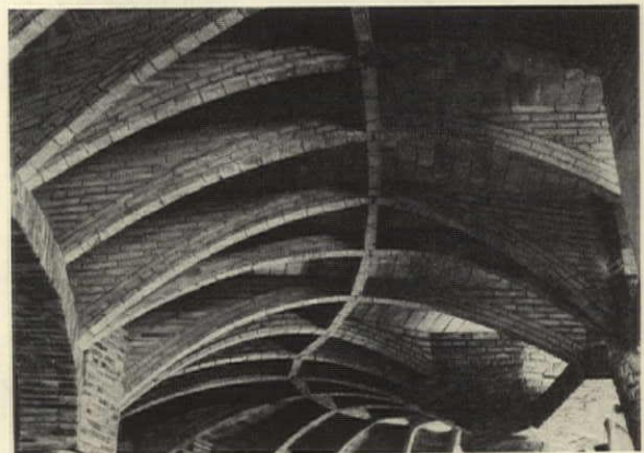
Vaulting in Güell Colony Chapel (1898-1914). Note thin masonry ribs
