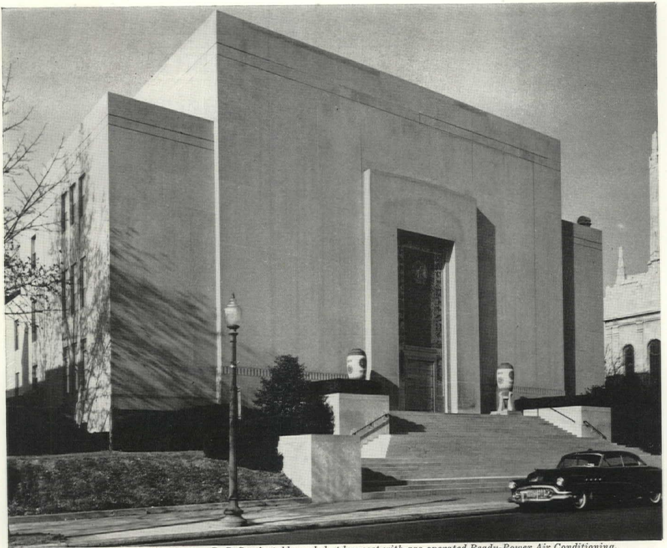
Scottish Rite Temple, Washington, D. C. Comfortably cooled at low cost with gas-operated Ready-Power Air Conditioning. Consulting Engineer: Silver Associates. Contractor: Joines Refrigeration, Inc.
