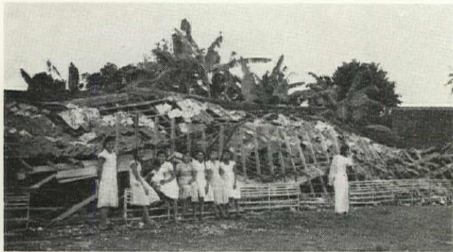
The temporary school buildings erected by a local contractor for the Christian Teachers College at Salatiga collapsed a few minutes after classes were dismissed
