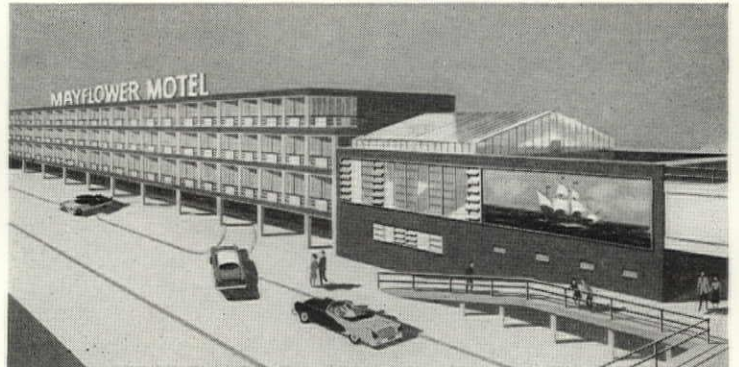
MAYFLOWER MOTEL, ATLANTIC CITY: Architect S. L. Malkind states: "In addition to being 25% cheaper than comparative materials, the happy union of prestressed concrete girders and floor beams and concrete columns provides a perfect foil for architectural decoration." This three-tiered motel was designed and built, from ground-breaking to opening, in five months. Architect: Samuel Lewis Malkind, New York, N. Y.; Consulting Engineer: Stresscon Associates, Newark, N. J.; Contractor: Ramat Construction Company, Spring Valley, N. Y.; Fabricator of prestressed elements: ATLANTIC PRESTRESSED CONCRETE COMPANY , Subsidiary of Warner Company, Trenton, N. J.
