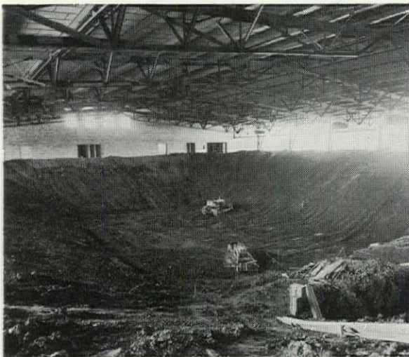
As shown in the photos, this unique design provides for excavating and pouring the bleachers on the earth as framework. The roof is supported at grade line by trusses incorporating haunches for support as an integral unit, without need for supporting columns. Spectator entrances and exits are at grade level. Seating capacity, 9,252. Building contains 81,555 sq. ft., with a construction cost of $10.41 per sq. ft.
