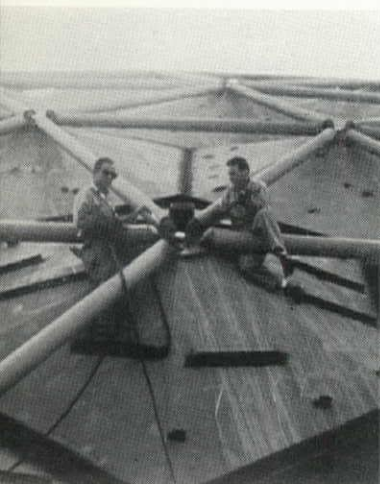
3 The hexagonal panels are 11-gauge hot-rolled sheet steel, ranging from 12' to 17" across; the struts are 6" schedule 10 steel pipe. All are welded together
