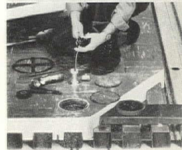
Service outlets can be installed anywhere on the floor. They can be relocated or new ones added — or circuits can be changed — without costly alterations.
