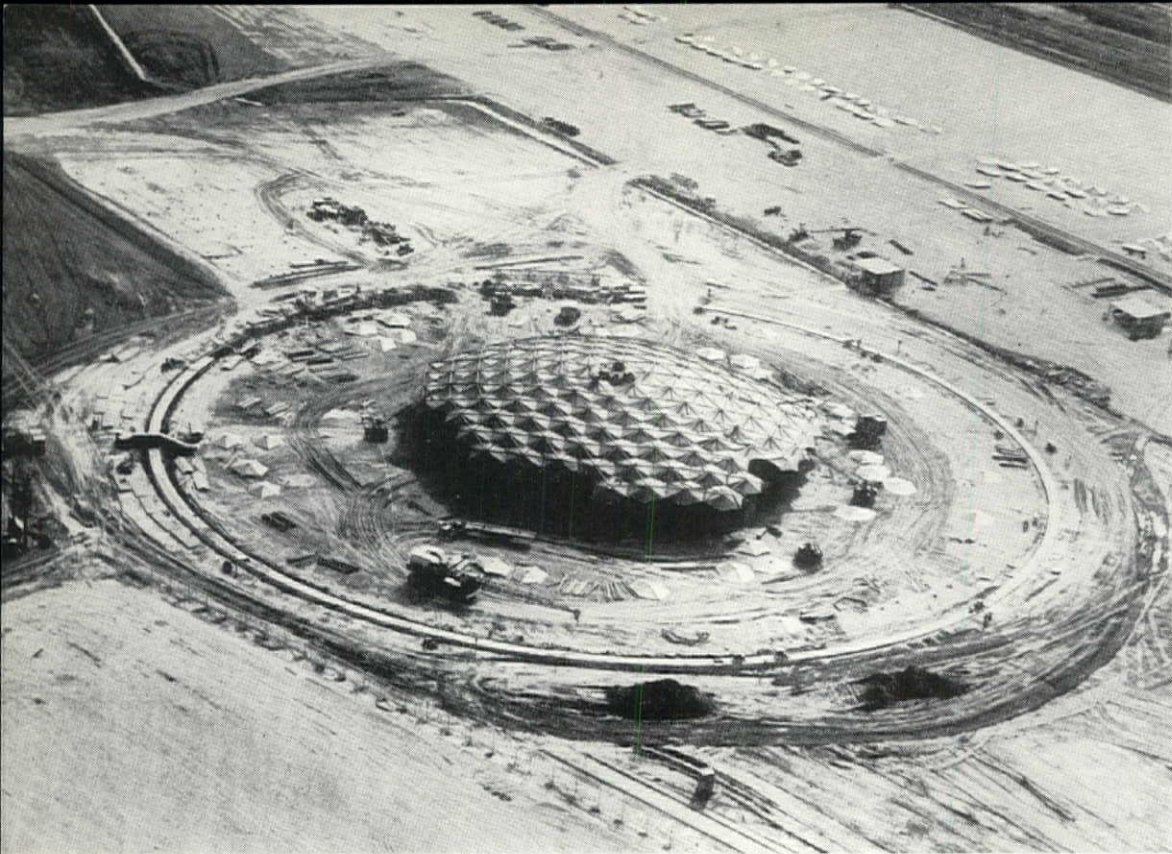
1 First portion of dome was erected on scaffolding 30' high. Outer ring is foundation, showing ultimate diameter
