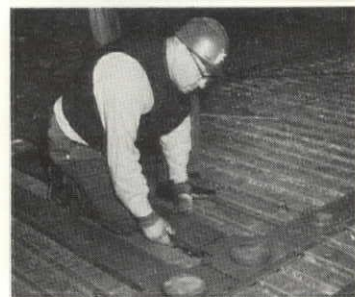
Service outlets can be installed anywhere on the floor. They can be relocated or new ones added — or circuits can be changed — without costly alterations.
