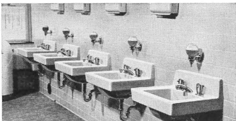
Briggs Milton Lavatories specified for Sacred Heart Academy are of fine vitreous china in two sizes, 24"x20" and 20"x18", for 8" combination fittings. 4 colors were used.
