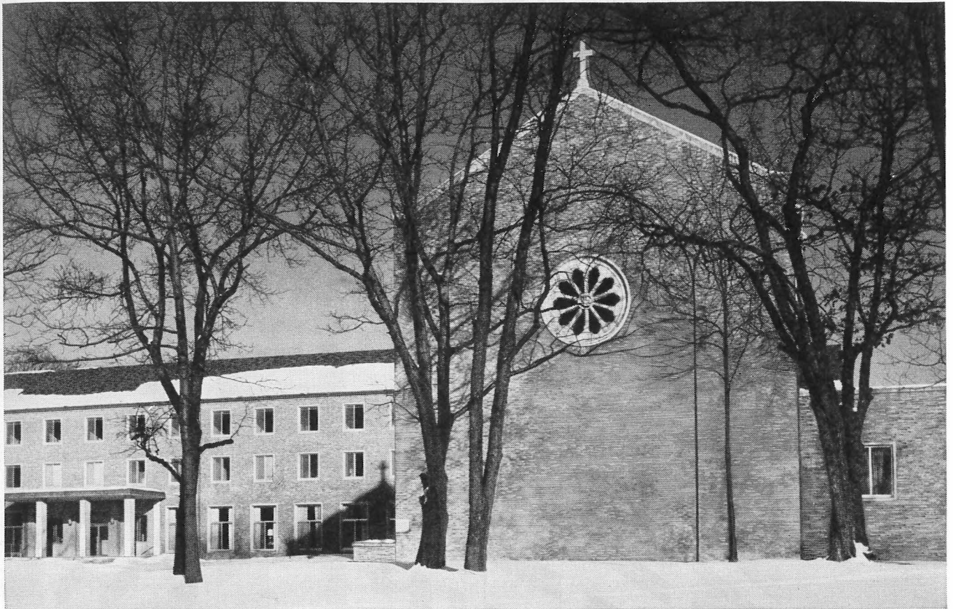
CONVENT AND ACADEMY of the SACRED HEART, Bloomfield Hills, Mich. Architects: Smith, Hinchman & Grylls Associates. Plumbing Contractors: Harrigan & Reed Heating & Plumbing Co.
